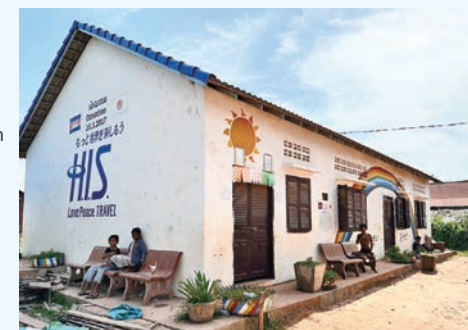
Elementary School built
